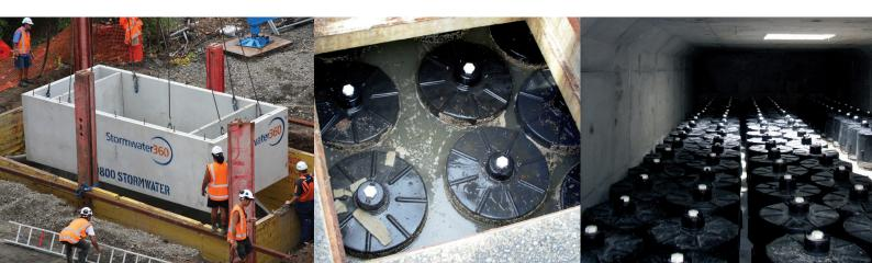
This revolutionary stormwater quality device is the latest in filtration technology and uses gravity, flow rotation, and up-flow membrane filtration to provide stormwater treatment in an underground compact stand-alone system.
