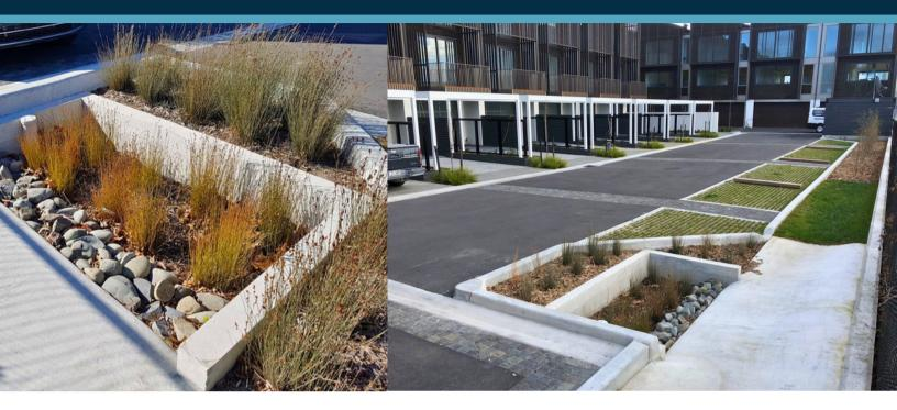
The first Filterra® installation in the South Island, the 2017 Fletcher development required a biofiltration device with a small footprint to treat 1,100m², and include infiltration. This custom Filterra® was the solution.
