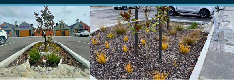
The <u>Filterra®</u> is a high infiltration, small footprint biofiltration system. Stormwater360 worked closely with the design consultants to create a bespoke design using a swale for conveyance and distribution, and an extended storage infiltration layer.
