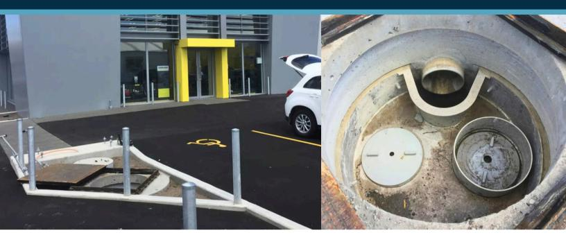
An innovative solution was required to treat 1150m<sup>2</sup> of impervious catchment in a commercial carpark development, a site with a low 229mm driving head.
