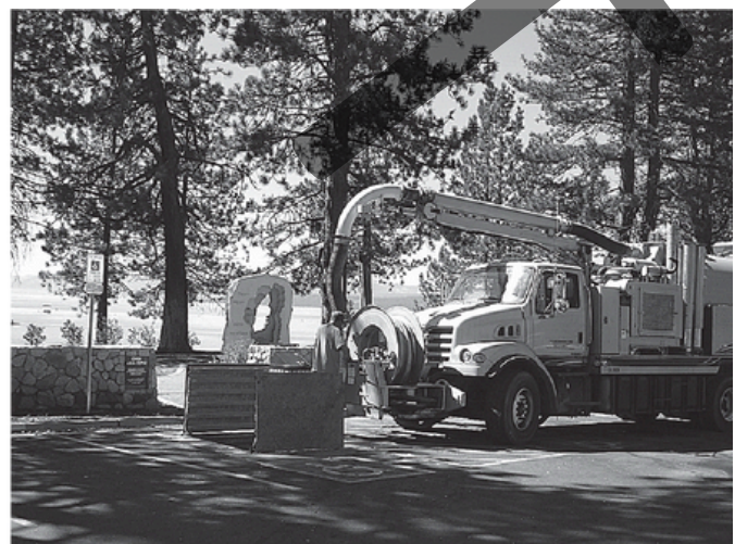
A vacuum truck removes pollutants from the system
