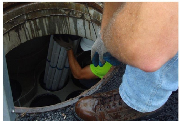
A view of a Jellyfish Filter cartridge deck from the surface showing all the cartridge lids intact and no standing water on the deck (left image), and inspection of the flexible separator skirt from inside the maintenance access wall opening (right image).
