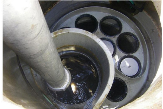
A maintenance worker stationed on the surface uses a vacuum hose to evacuate water, sediment, and floatables from the Jellyfish Filter by inserting the vacuum wand through the maintenance access wall opening.
