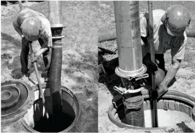
A maintenance worker stationed on the surface uses a vacuum hose to evacuate water, sediment, and floatables from the Jellyfish Filter by inserting the vacuum wand through the maintenance access wall opening.
