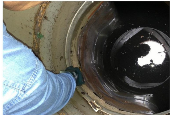
A view of a Jellyfish Filter cartridge deck from the surface showing all the cartridge lids intact and no standing water on the deck (left image), and inspection of the flexible separator skirt from inside the maintenance access wall opening (right image).
