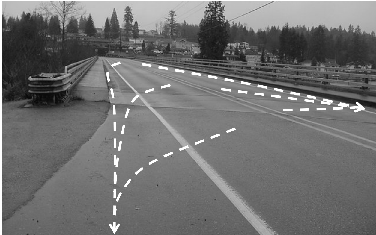
Figure 4. View of part of the Lake Stevens North StormFilter site drainage area. Arrows indicate flow to the StormFilter system via gutters and catchbasins located at the foot of the bridge.
