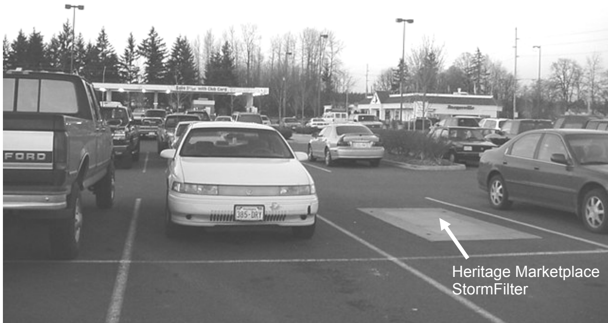
Figure 2. View of part of the Heritage Marketplace StormFilter site drainage area in proximity to the StormFilter.
