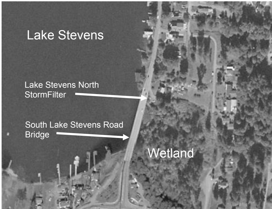
Figure 3. Aerial view of the Lake Stevens North StormFilter site.
