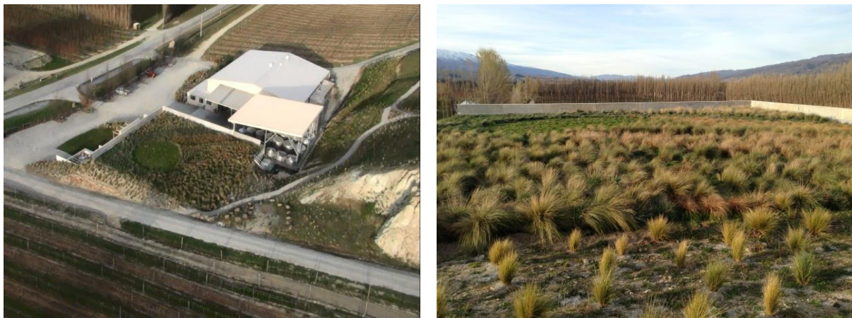
Figure 6: Mt Difficulty living Roof
