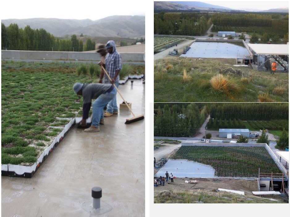
Figure 7: Mt Difficulty living roof Installation
