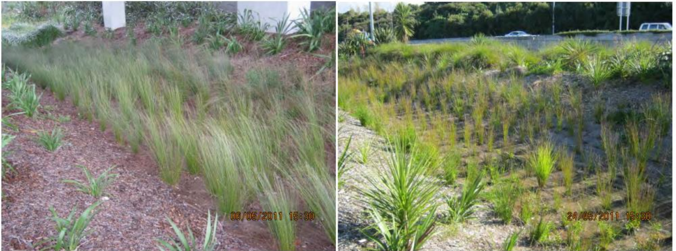
Figure 5 – Examples of vegetated swales for the treatment of road runoff (State Highway 1, Auckland)
