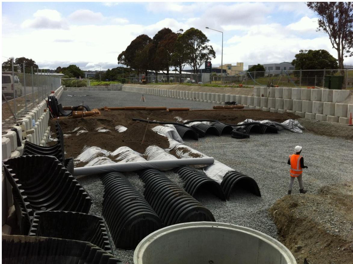
Figure 1: Bioretention Device during Construction
