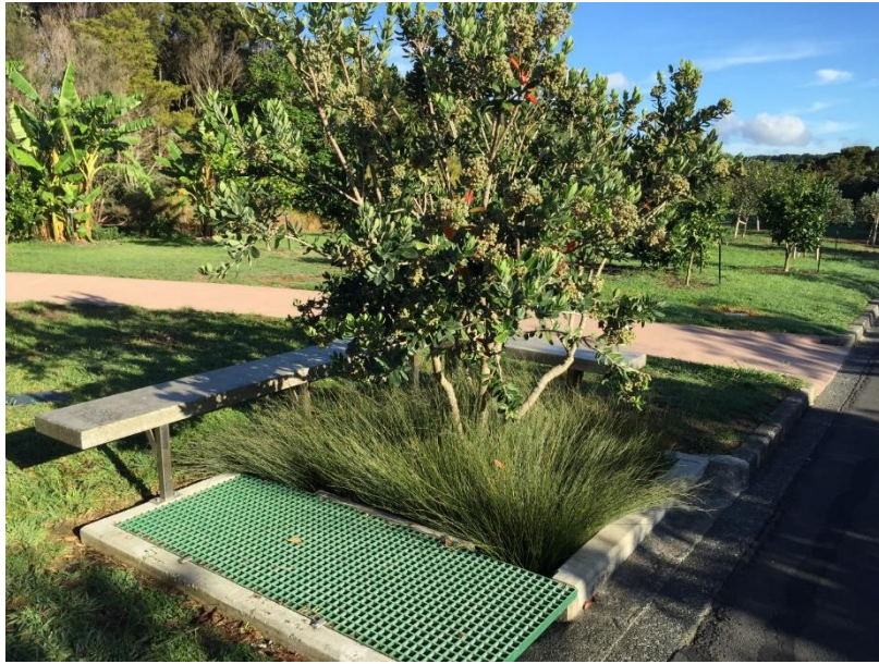
Figure 1 BioFilter stormwater treatment device at Auckland Botanic Gardens, June 2015 (approximately aged three years)
