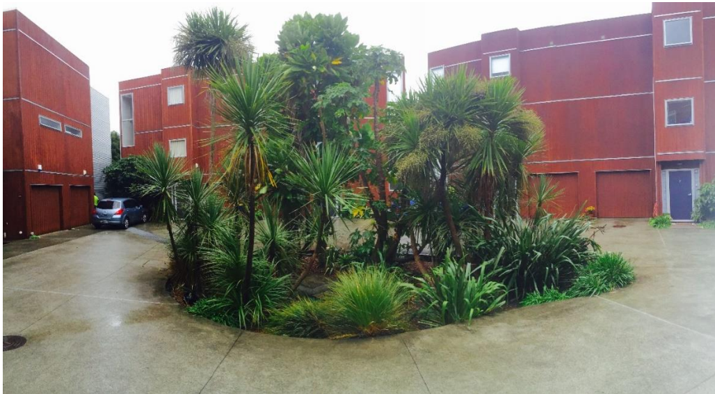
Figure 7: Photo of Raingarden/Proprietary Media Filtration Cartridge hybrid treatment train at Henderson, Auckland (Source: Stormwater360 NZ)
