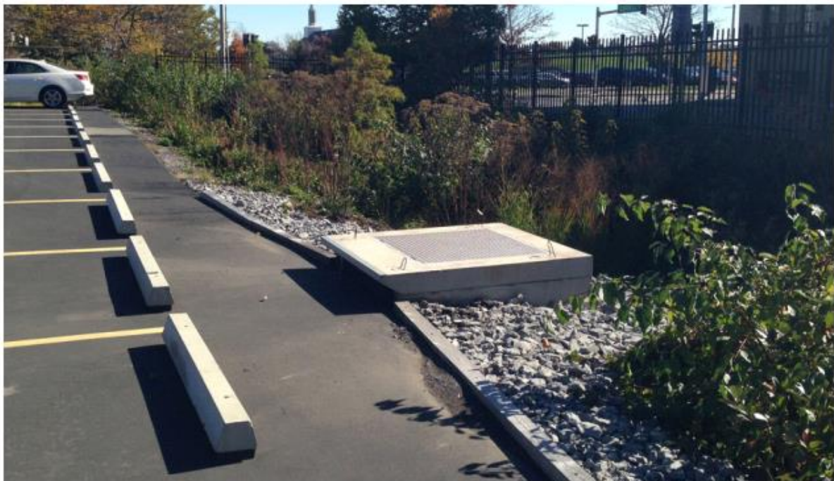
Figure 8: Photo of Hybrid treatment train at Buffalo Niagara Medical Campus (Source: Contech Engineered Solutions)
