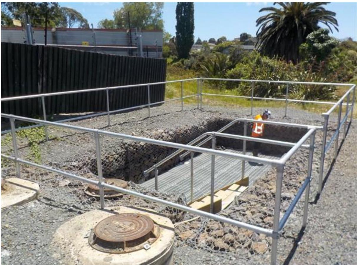
Figure 9: Handrails installed on StormFilter Retrofit (Source: Stormwater360, 2016)
