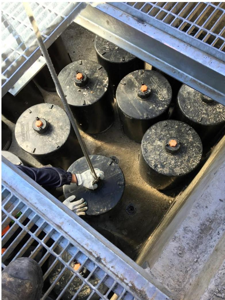
*Figure 6: Installing StormFilter Cartridges (Source Stormwater360, 2016)*
