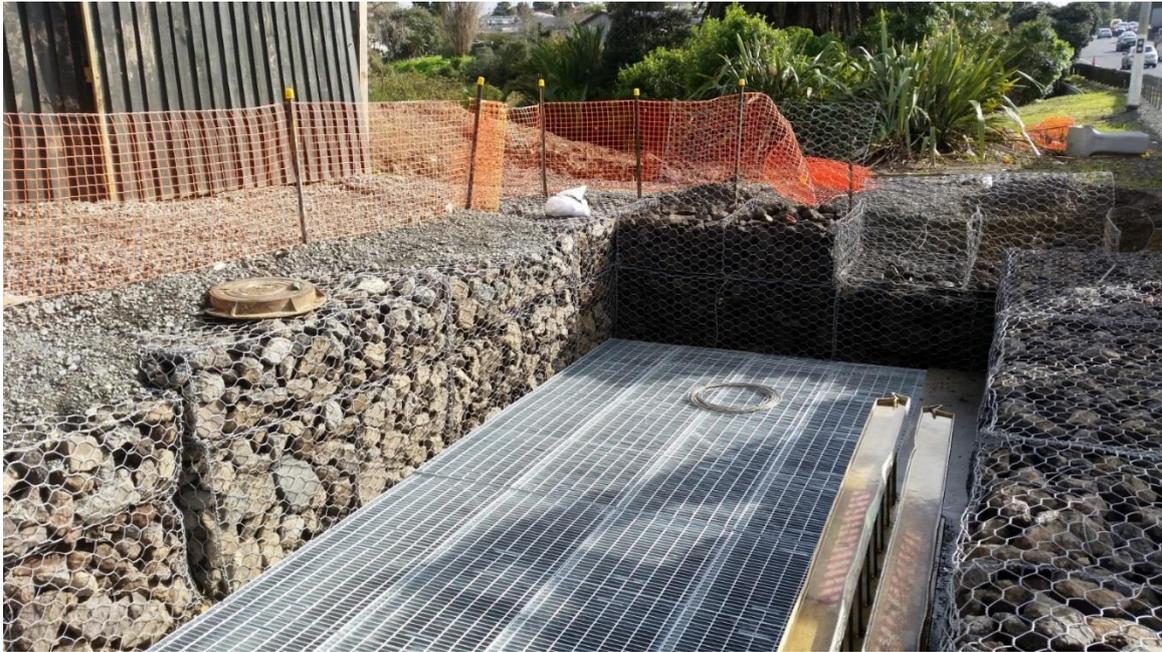
Figure 8: Grated top of StormFilter Retrofit (Source: T Brockbank, 2016)
