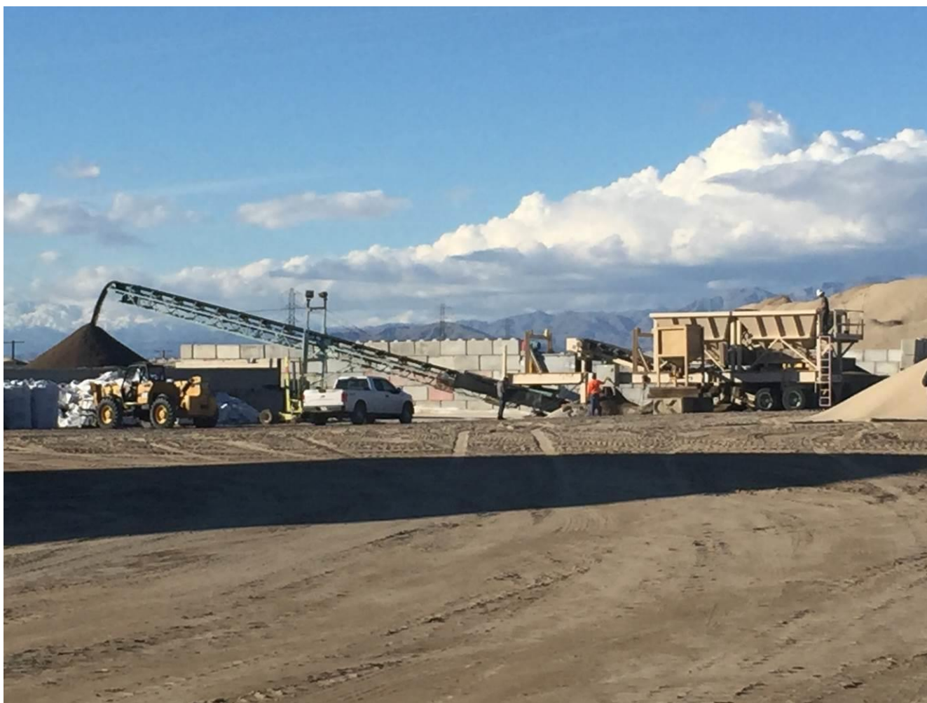
Figure 3 Pug mill used to blend Contech Filterra rapid bioretention media
