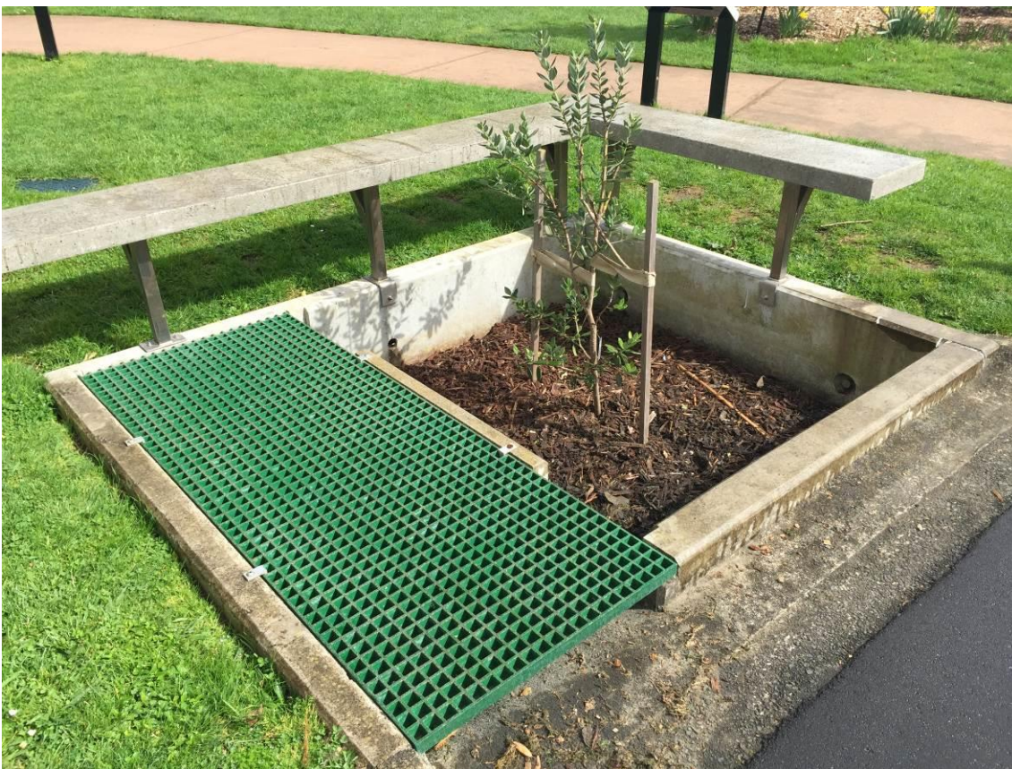
Figure 4 Filterra rapid bioretention device at the Auckland Botanic Gardens
